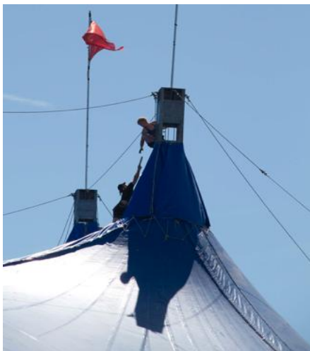
Fig EK 5. install of bale-ring cover.
